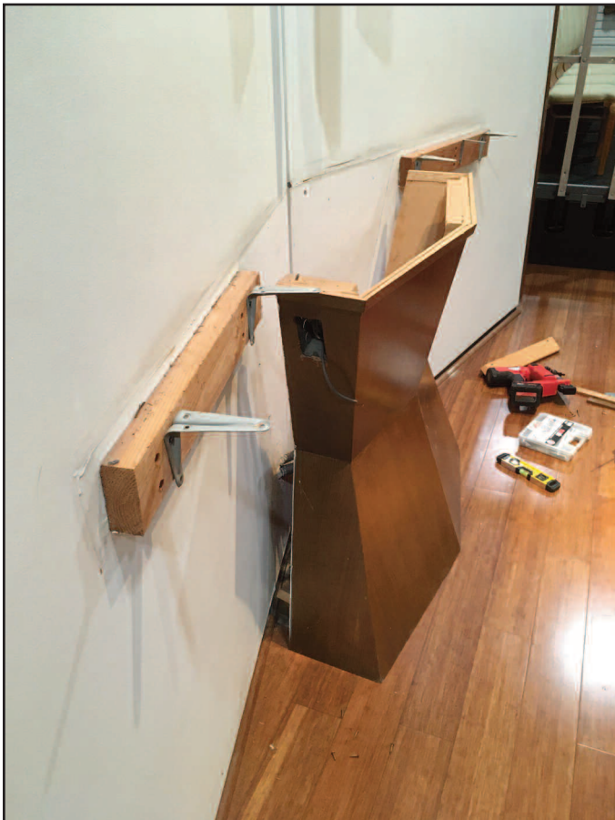
Altar being repaired
