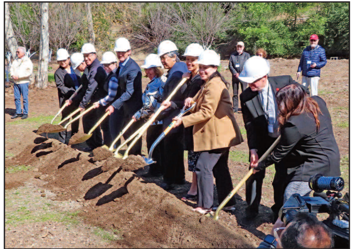
The ground is broken and construction is underway.
