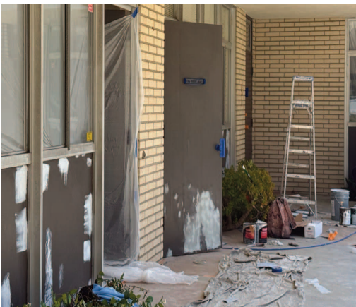
Repainting in progress
